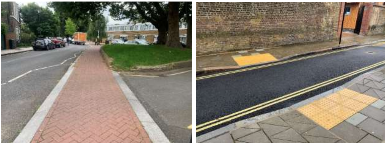
Figure 7-6: Continuous footway provision (Left – Claylands Road) and Dropped kerb with tactile paving (Right – Sans Walk)
