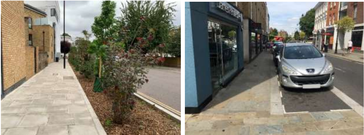
Figure 7-5: Example of clear footway space incorporating SUDs (Left – Crossway) and Recessed loading pads enable footway widening in constrained streetscapes (right – Clapham Old Town)
