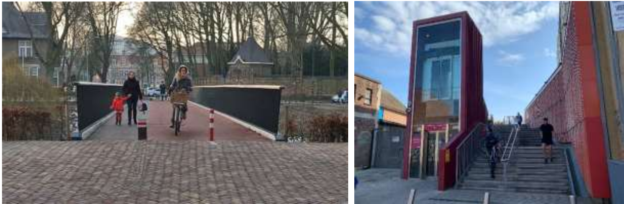
Figure 7-8: Example of a pedestrian + cycle bridge (Left – Mariabrug) and example of a new bridge incorporating access for steps, lift and ramps (Right – Wallis Road, Olympic Park)
