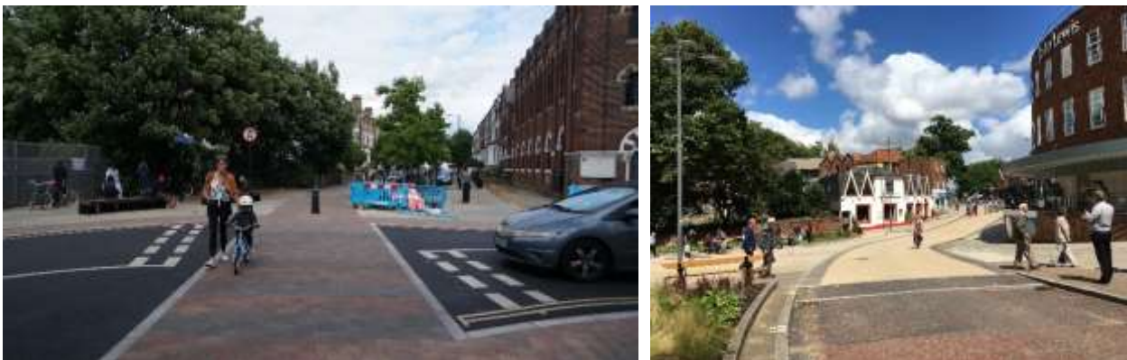
Figure 7-4: Implied crossing provides direct crossing on pedestrian desire line (Left- Downs Road), and example of a raised table crossing in Norwich (Left – Westlegate)
